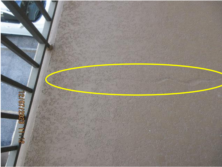
View of crack along walkway coating
