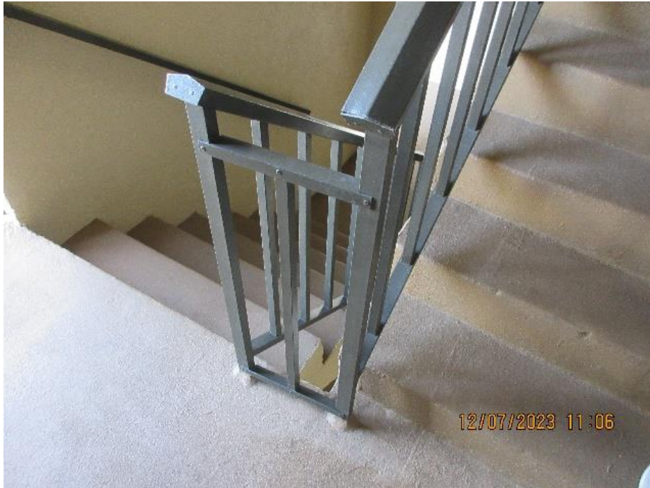
View of cored railings along stairwell
