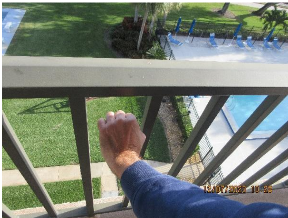
View of balcony railing picket spacing
