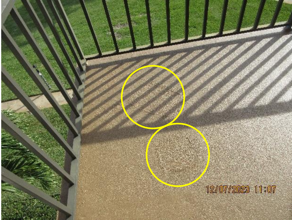
View of concrete patches on balcony slab
