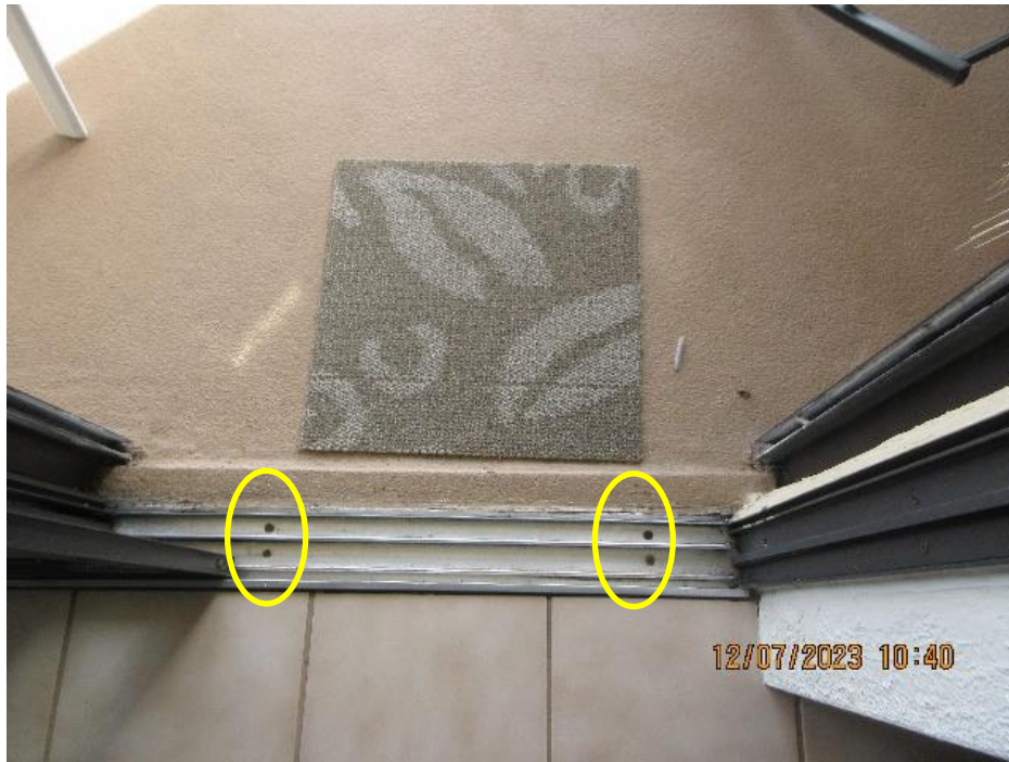
View of corroded fasteners at sliding glass door
