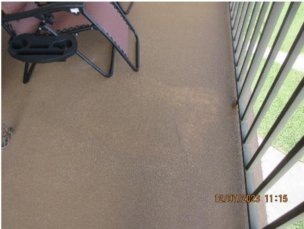
View of missing texture to balcony coating
