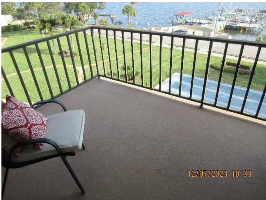
View of cored in place balcony railing
