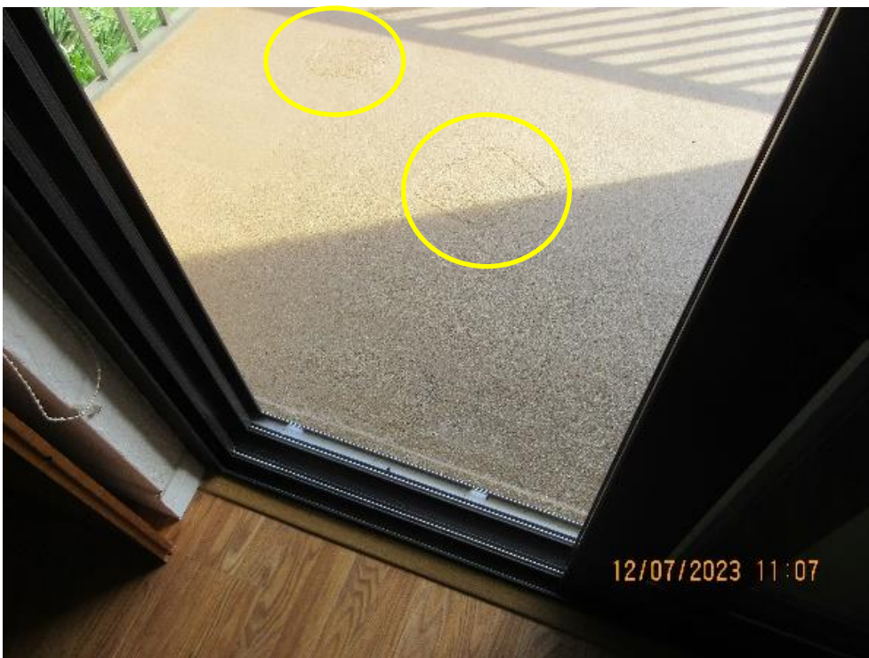
View of concrete patches on balcony slab
