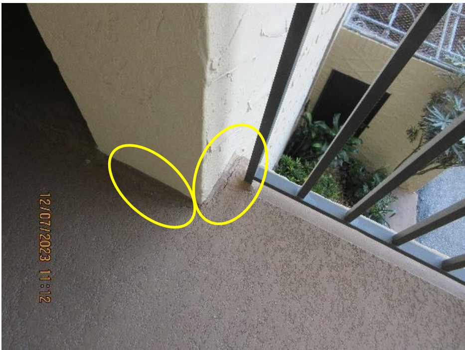
View of crack at floor to wall joint
