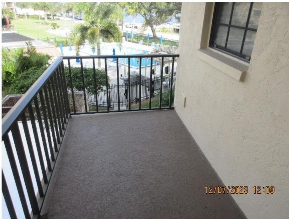
View of cored railings along walkway
