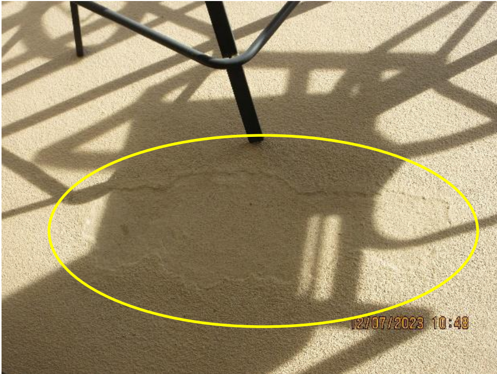
View of missing texture to balcony coating
