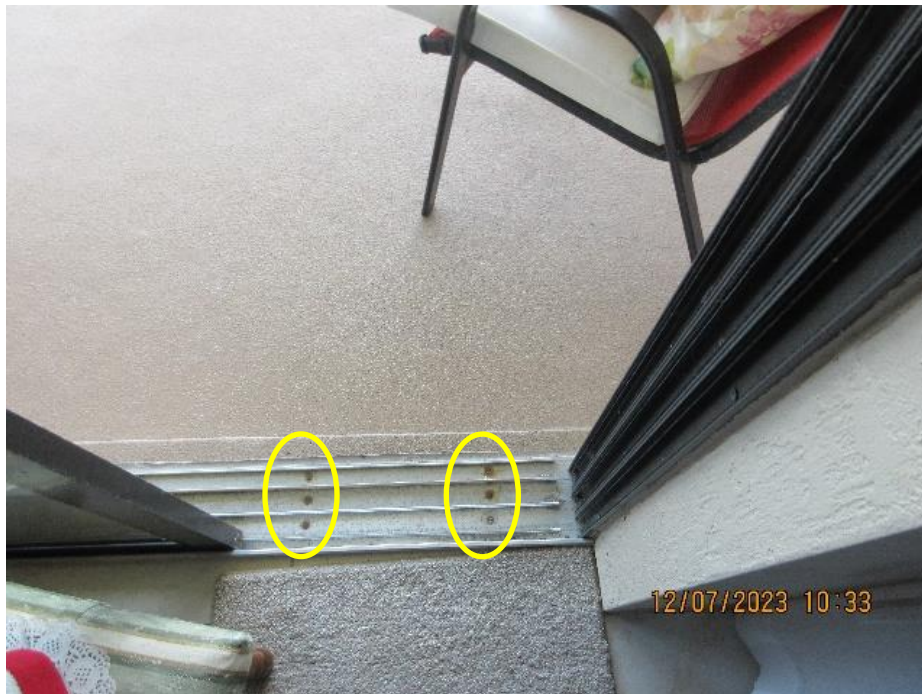
View of sliding glass door track with corroded fasteners
