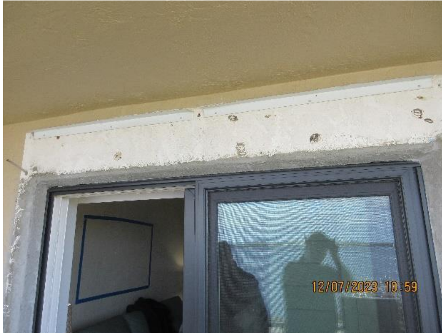
View of uncoated area under former shutter
